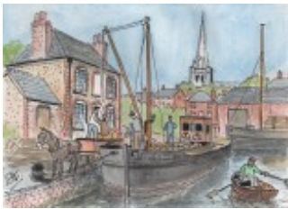
11. Chi Canal Wharf
